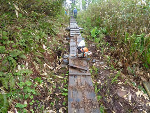
3-1 C・D地点補修前
